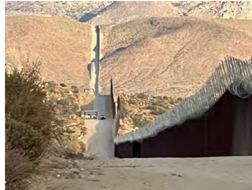
Figure 5. CBP vehicles patrol the only road leading to the Willows site. (Photo from November 14, 2023).
